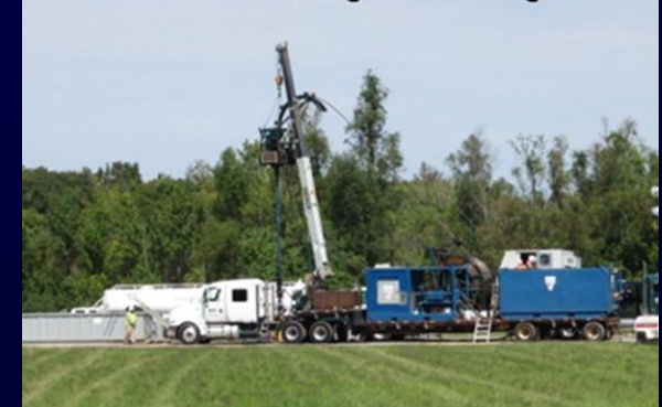
ORW #2 Well... Coil Tubing Unit Cleaning out Well
