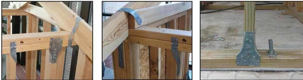
**Figures 6-15, 6-16 and 6-17.** In the LaHouse model home, hurricane straps are used to complete the continuous load path connection. The stud to single plate connector helps secure the house frame to its foundations and helps the home better withstand uplift. For new construction, the additional cost of implementing stronger connections may be minimal (Figures 6-15 and 6-16, photos by D. Hwang, 2007; Figure 6-17, photo courtesy of LSU AgCenter).
