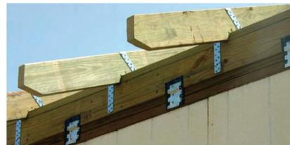
plate, which has anchors in the concrete walls. Framing lumber is secured to the rim band with hurricane straps. Soffits and soffit vents made of perforated fiber cement will be attached securely to framing members.
