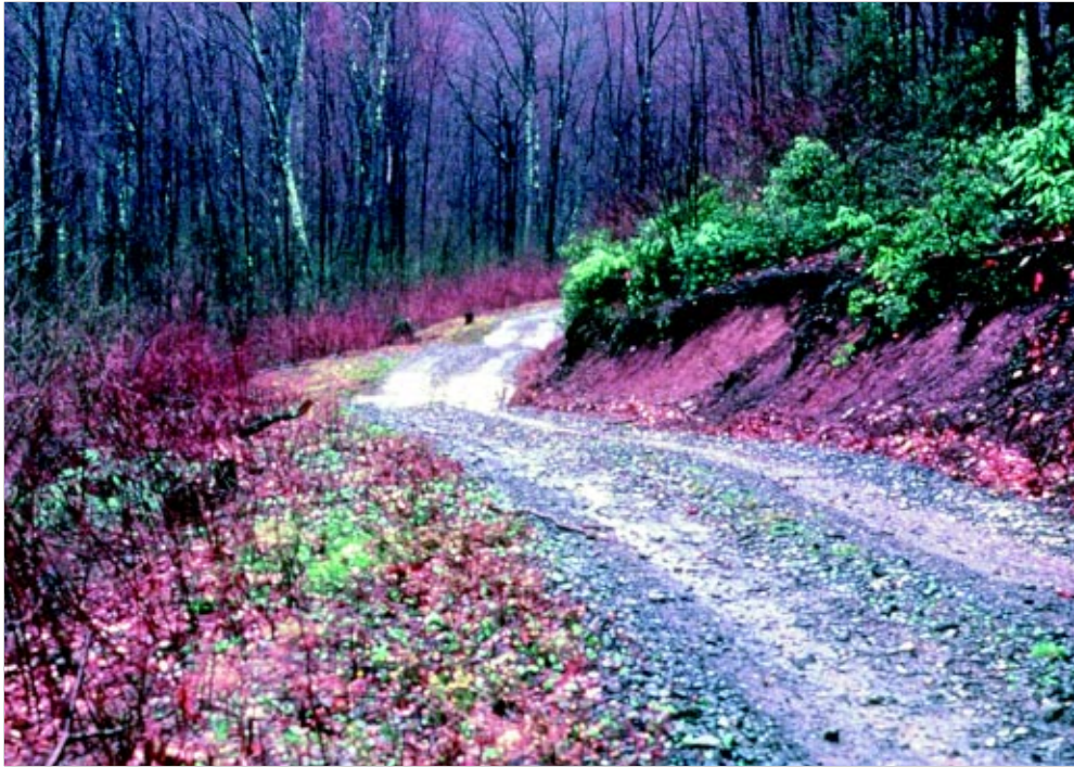
An example of rolling dips on a permanent road.
