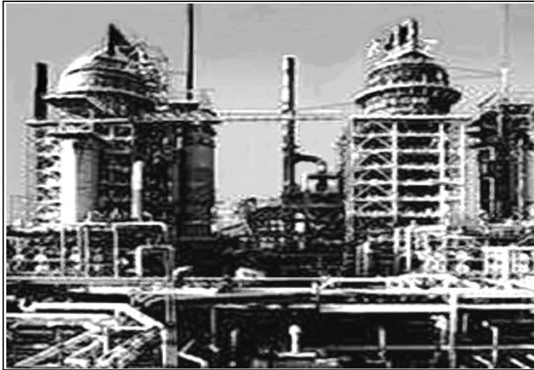
Exxon-Mobil Refinery - Baton Rouge
