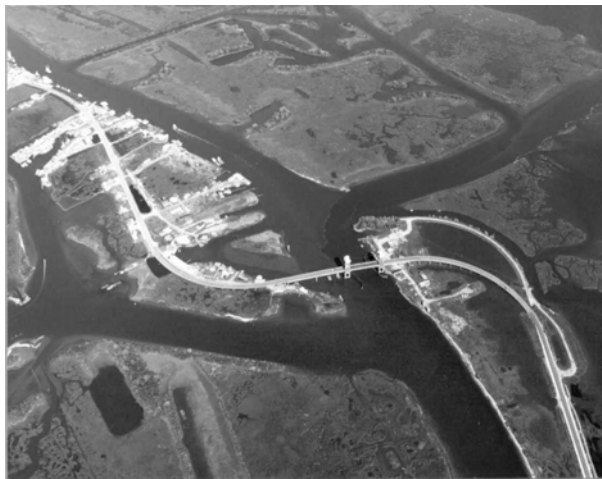
Leeville Bridge the "weakest link" in the supply chain to Port Fourchon.
