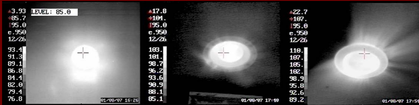
Unsealed down lights & leaking escutcheons
