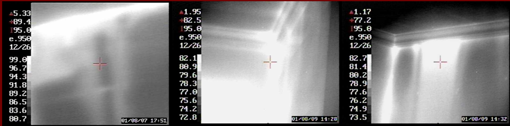
Insulation voids and leaking top plate.
