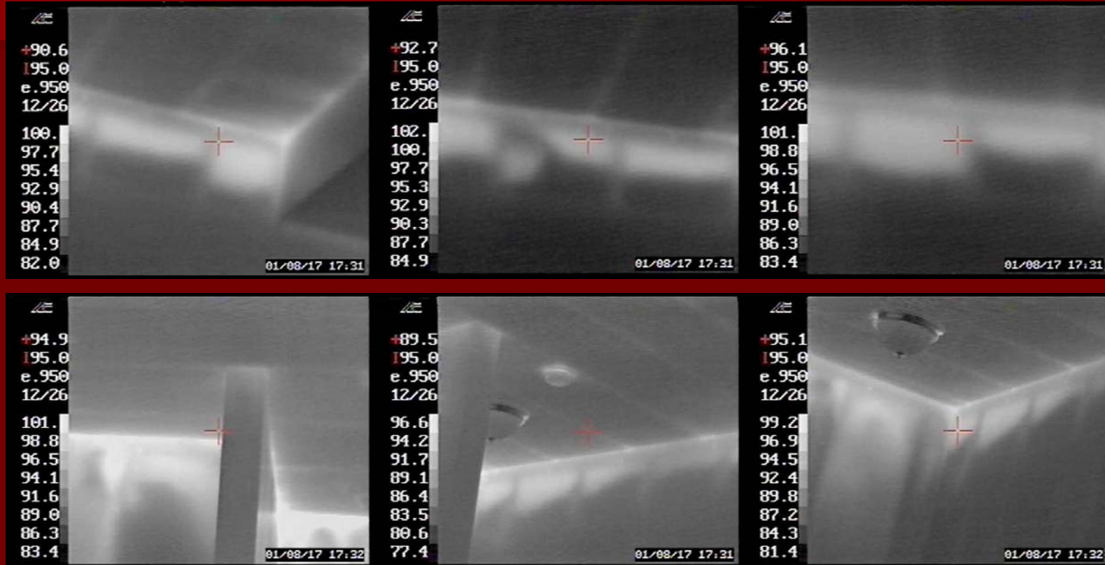
Hot spots from voids at the top of the walls in the Great Room.
