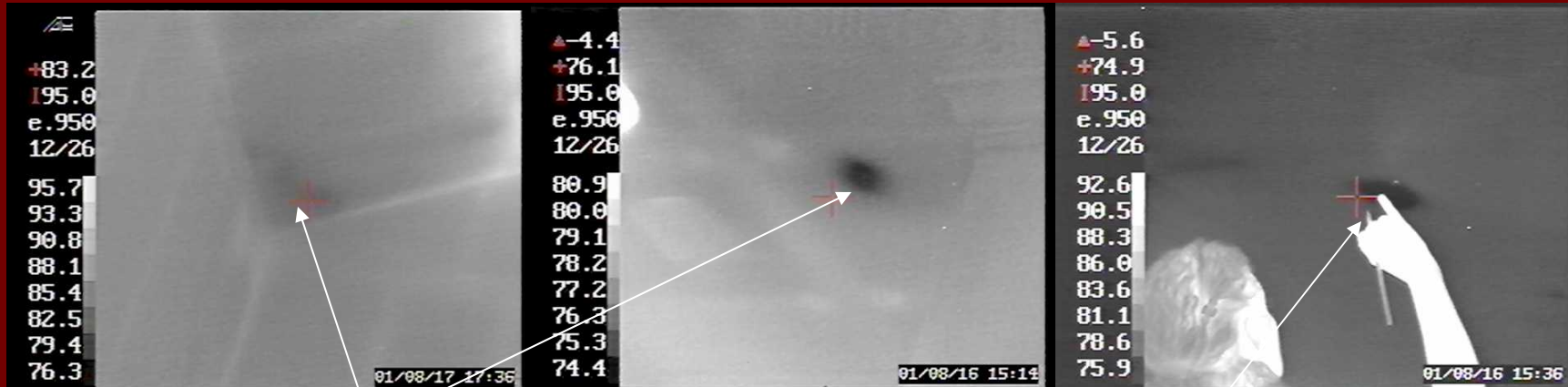
Roof leaks showing from evaporation pattern in ceiling.
