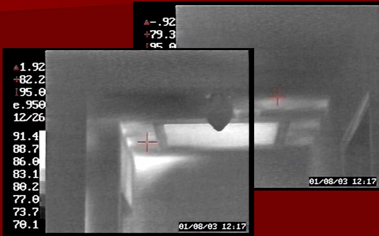
Overlapping images show the extent of voids in a hallway around an non-insulated stair hatch.
