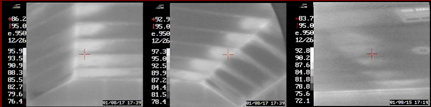
Poorly distributed blown insulation
