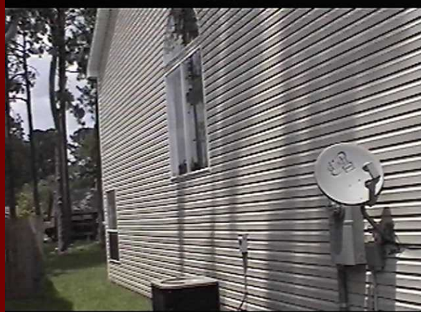
Vinyl siding leaks unmasked.
