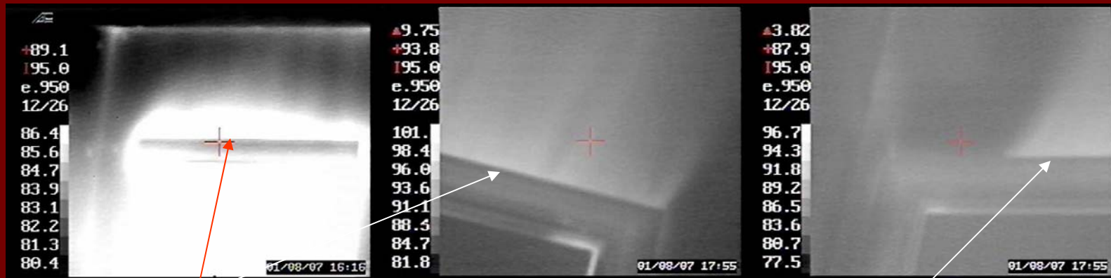
Air leaks at window and door frames from poor caulking jobs.
