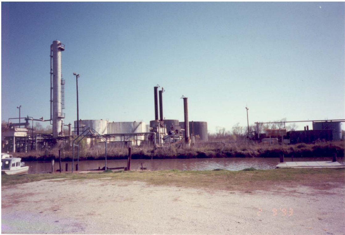
Cameron Resources Refinery, taken in Feb 93
