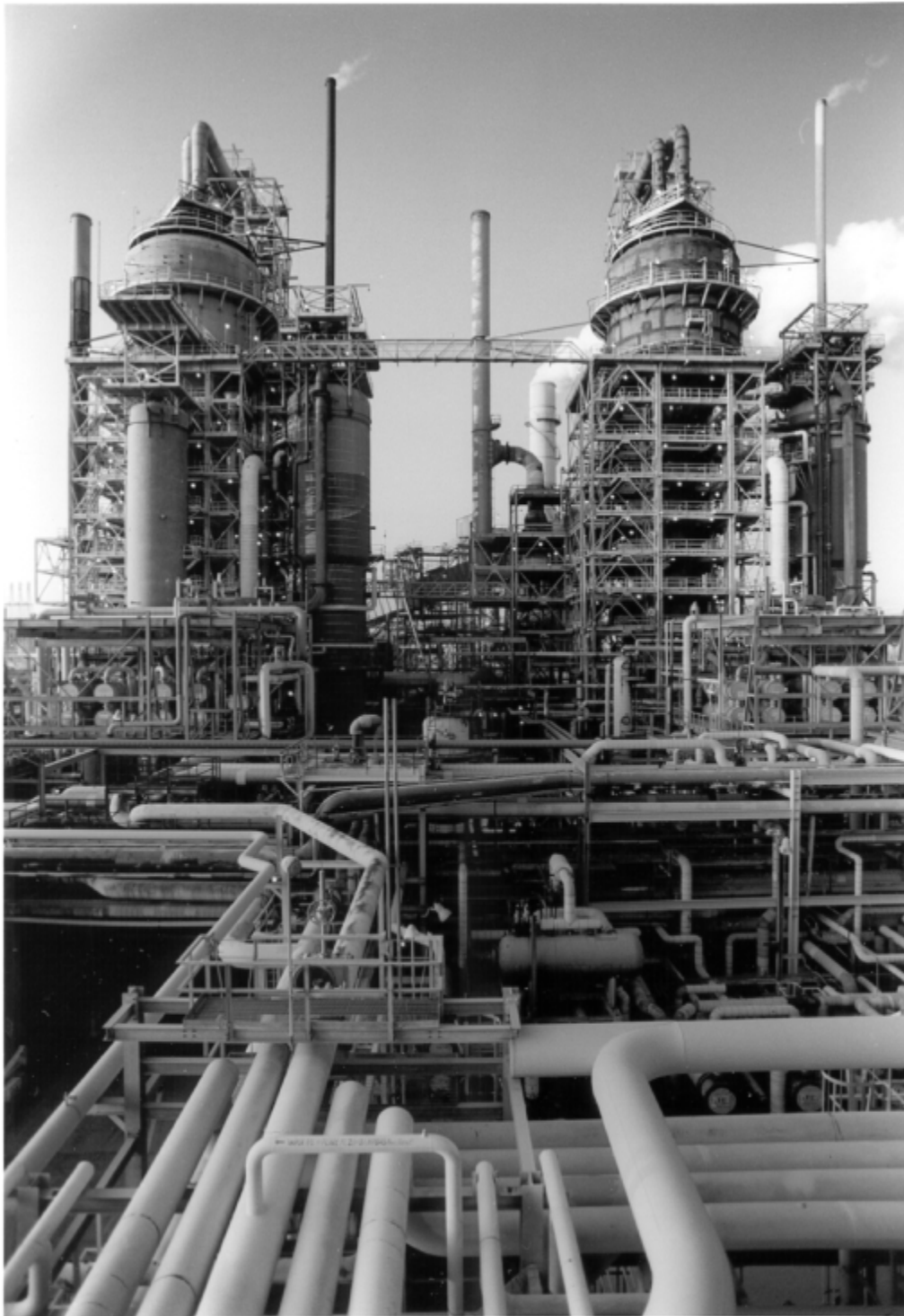
Catalytic-cracking technology, invented at Exxon Baton Rouge in 1942, helped win WWII. It remains an industry standard. Photo courtesy Exxon Public Affairs.
